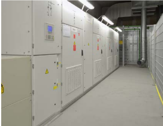
Caption: The POCOS-S reactive power compensation systems, which can be switched in stages, has optimized costs at Alunorf. The compact systems with a modular cabinet design are used in the 6 kV medium voltage grid.
