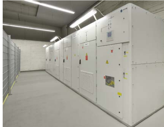
Caption: The POCOS-S reactive power compensation systems, which can be switched in stages, has optimized costs at Alunorf. The compact systems with a modular cabinet design are used in the 6 kV medium voltage grid.
