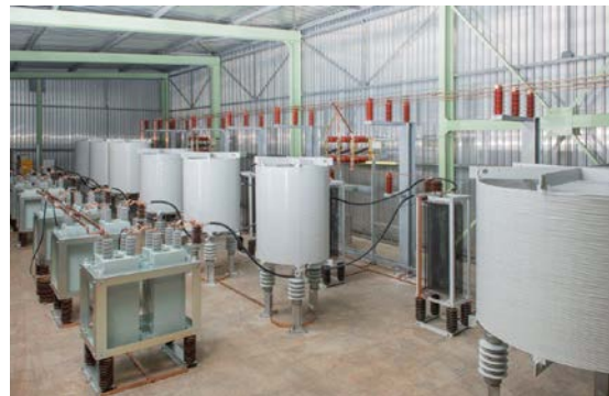
Caption: The 30 kV filter circuit system from MR has achieved optimized and economical power distribution while improving reliability of production and supply at the same time.
