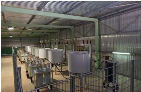
Caption: The 30 kV filter circuit system from MR has achieved optimized and economical power distribution while improving reliability of production and supply at the same time.
