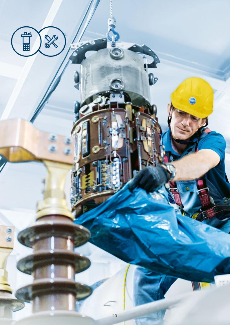
The on-load tap-changer is the most important component in a regulated transformer. Maintenance and care of this highly accurate device is thus of utmost importance. With TESSA® Premium Service, we ensure the reliable and state-of-the-art operation of the on-load tap-changer for the whole lifetime of the transformer. Globally and also for non-MR products."
