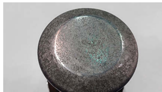
Fig. 20: RMV-II 2500 A vacuum interrupter contact after 1.8 million EAF-operations
