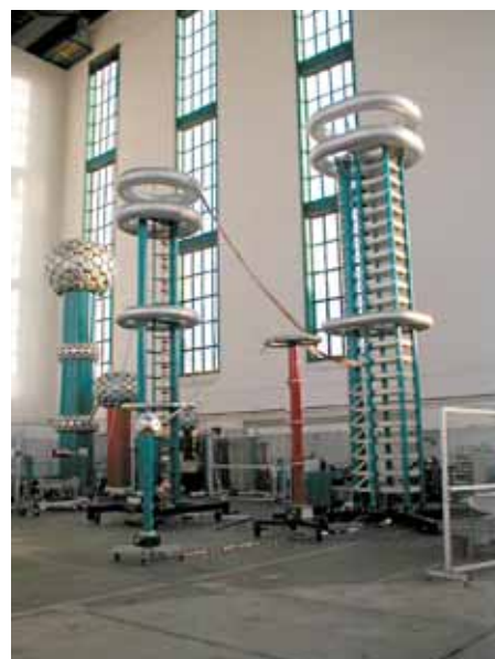
Calibration of an impulse voltage measuring system
